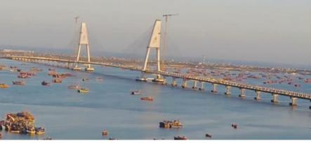
including 900 metres of central double span cable-stayed portion and a 2.45-km-long approach road, has been constructed at a cost of Rs 979 crore, as
