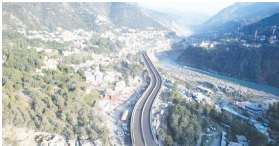
way-44. Gadkari said this extraordinary viaduct is composed of 26 spans and employs a combination of concrete and steel girders in its structural design. Its completion significantly alleviates traffic congestion in Ramban Bazar, facilitating the smoother flow of vehicles, he added.
