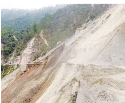
SHILLONG, Aug 26 (Agencies): A mudslide caused by incessant rainfall blocked the Sonapur tunnel on NH 6 in Meghalaya's East Jaintia Hills district
